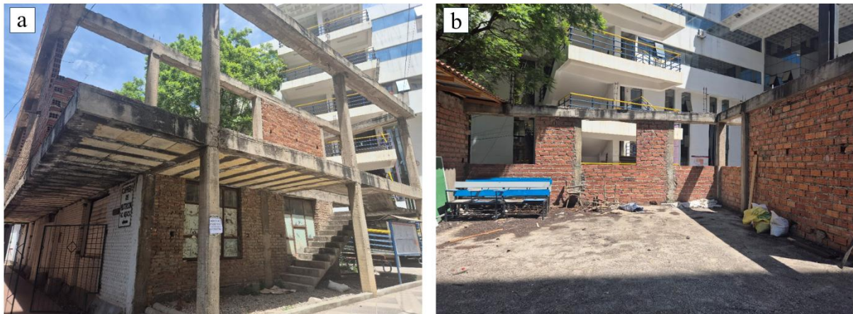
Figure 5. (a) General view and (b) upper floor of the building.
