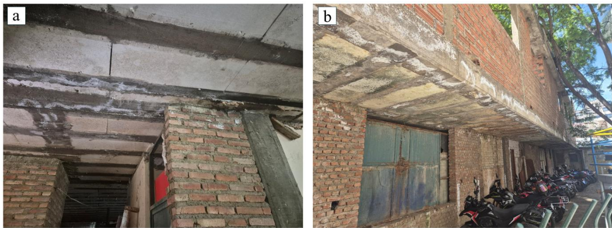
Figure 6. Underside of: (a) slab and (b) cantilever.
