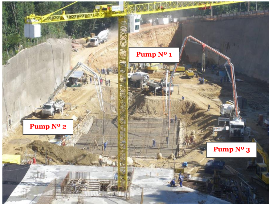
Figure 10. General view – Concrete pumps positioned.
