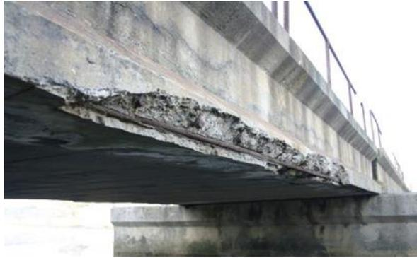
Figure 1. Corrosion-induced damage on a concrete bridge exposed to air-borne chlorides close to the shore in Cape Town
