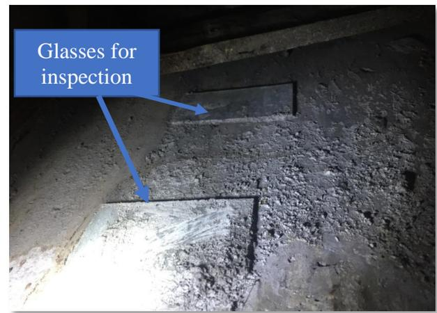
Figure 15. Interior of inspection window.
