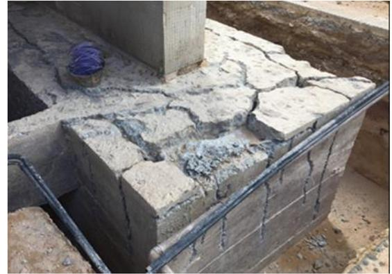
Figure 8. Cracks on a block with AAR.
