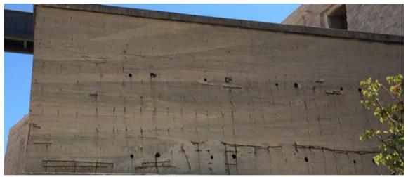
Figure 3. Carbonation-induced corrosion in areas of poor or inadequate concrete cover.
