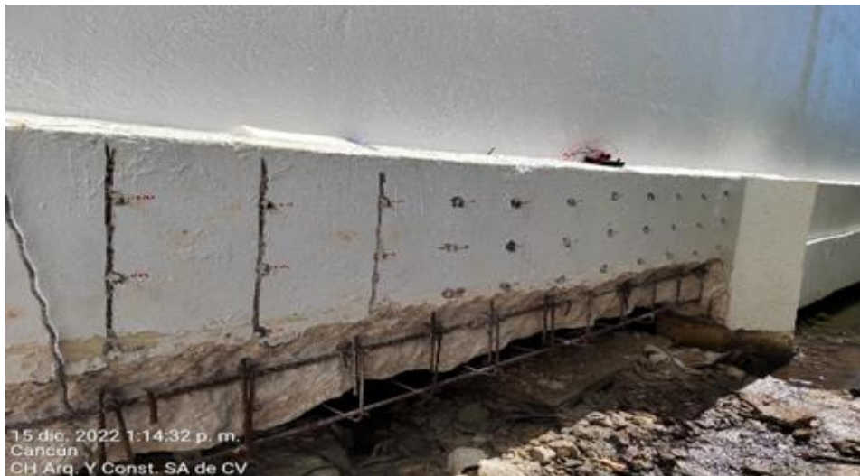
Figure 16. Installation of anodes inside host concrete with installation verification in Cancun, Mexico.
