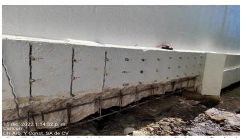
Figure 16. Installation of anodes inside host concrete with installation verification in Cancun, Mexico.
