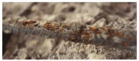
Figure 5. Typical pitting chloride induced corrosion.
