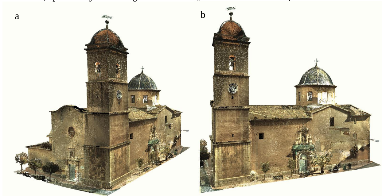
Figure 1. Main facades of the church obtained by topographic survey with Laser-Scanner. (a) Main entrance, (b) Facade of San Pedro.
