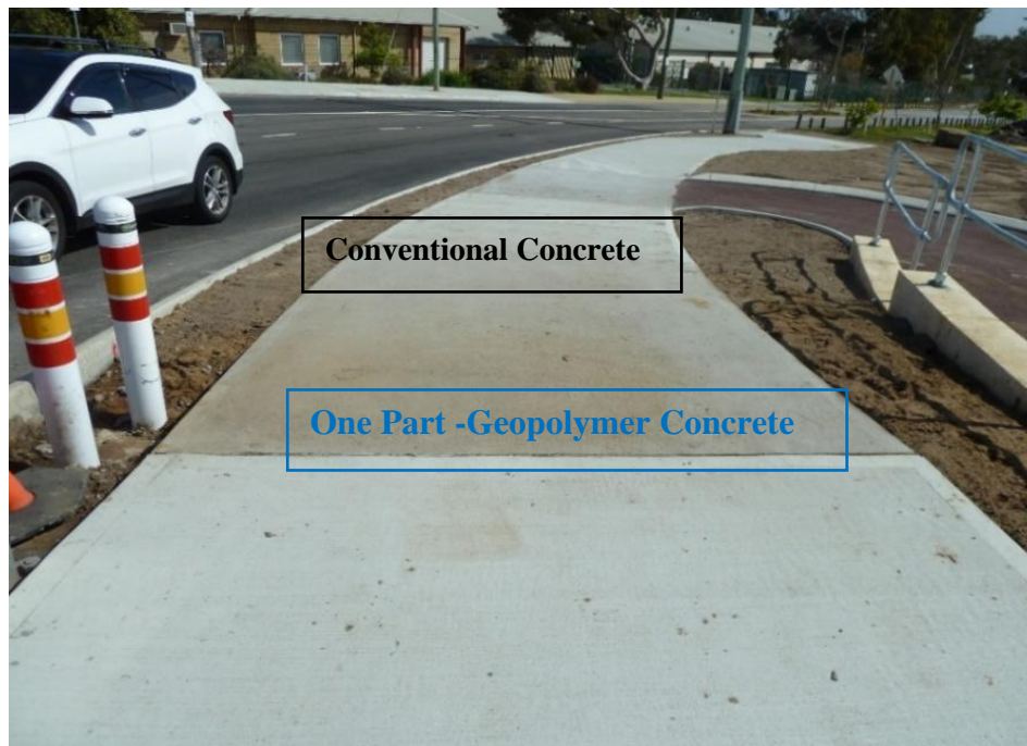
Figure. 4. Dual Use Concrete Foot Path
